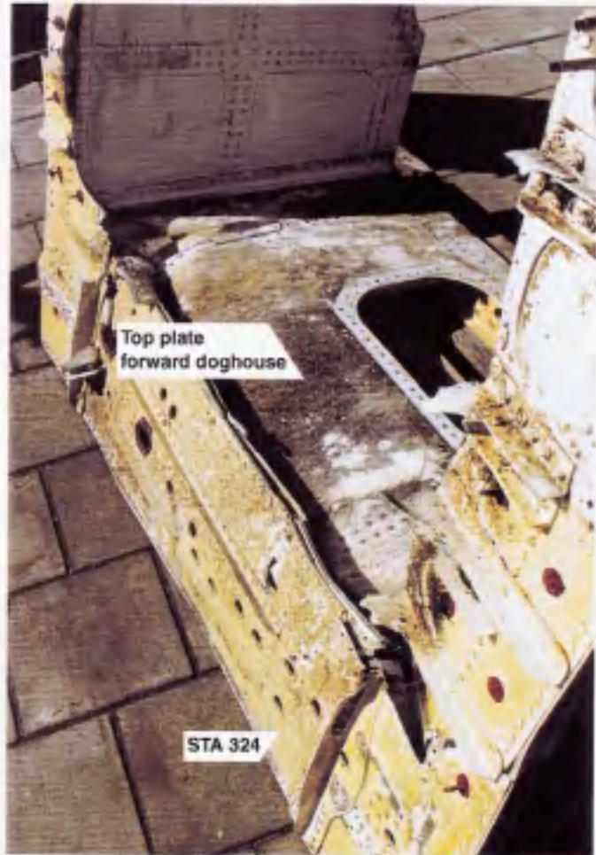
Fig. 6 Aft part of the forward doghouse and part of the STA 324 bulkhead (upside down position)
